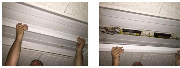
4. **Step 4:** Cut the leads from the ballast to the socket housing on both ends of the luminaire and cap socket leads. When cutting the leads, leave the smallest amount of wire attached to the luminaire.
