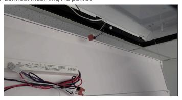
Flange Troffer Kit (TFD) Installation Instructions | Page 4 of 4 7. **Step 7:** Slide brackets through fixture slots, bend bracket over and secure with provided screws.
