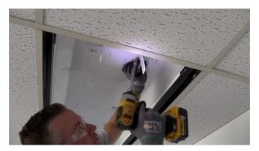
4. **Step 4:** Secure provided tether to existing fixture body.
