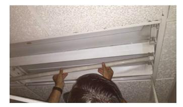
3. Step 3: Remove the wiring compartment cover. Set aside.
