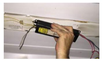
5. **Step 5:** Lamp Holders MUST be non-shunted, T-Series Medium Bi-Pin. A qualified electrician should assess the lamp holders for continued use or replace with new non-shunted lamp holders.
