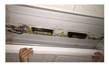
4. **Step 4:** Cut the leads from the ballast to the lamp holders on both sides of the ballast. When cutting the leads, leave the smallest amount of wire attached to the lamp holders as possible. Remove ballast from housing and dispose of properly.
