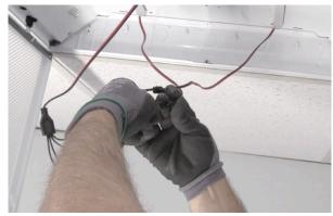
**Step 5:** Connect Driver DC 0-10V dimmable wire (when controls are being used), ground wire and AC connections.
