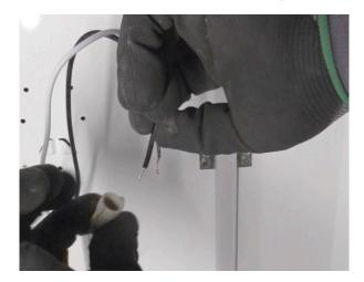
**Step 6:** Place belly pan cover over new driver and wiring.
