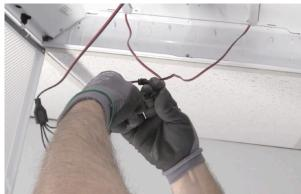
5. **Step 5:** Connect Driver DC 0-10V dimmable wire (when applicable), ground wire and AC connections.
